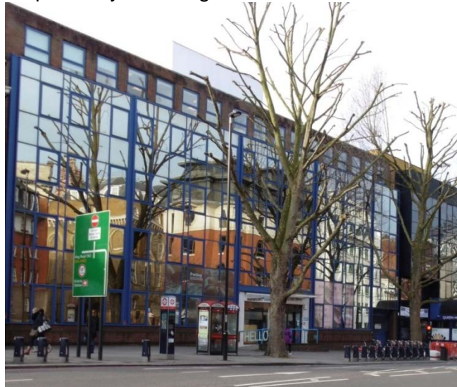
Figure 5.10 No.215 Vauxhall Bridge Road
