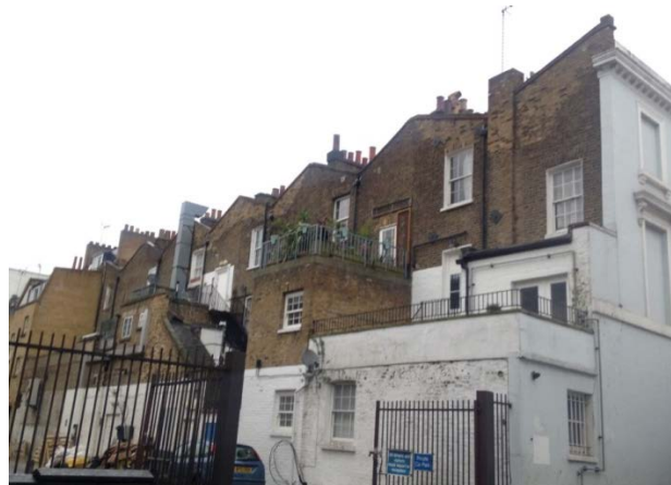
Figure 5.11 Nos.2-22 Upper Tachbrook Street
