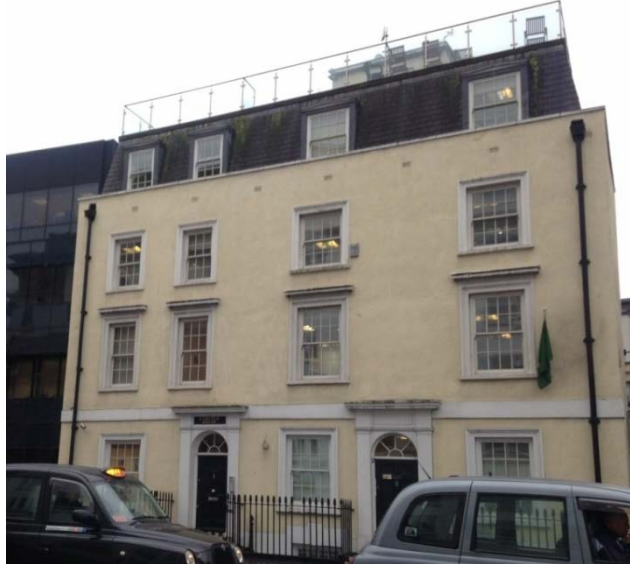
Figure 5.8 Nos. 235 & 237 Vauxhall Bridge Road
